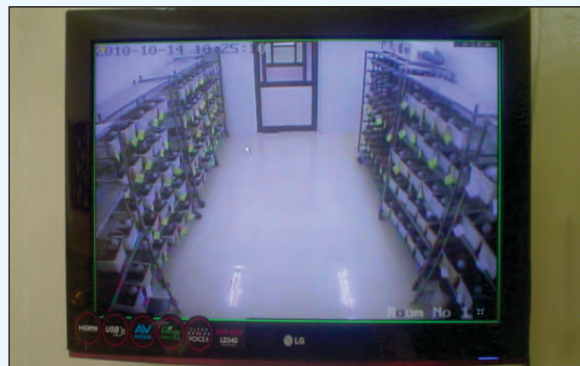
CCTV Camera (Room View)
